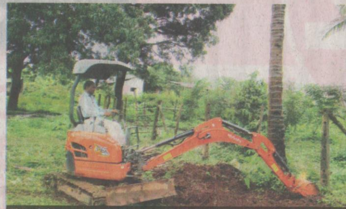
The mini-excavator at Don Bosco College of Agriculture, Sulcorna
